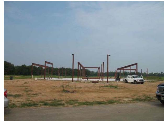
August – steel is going up
